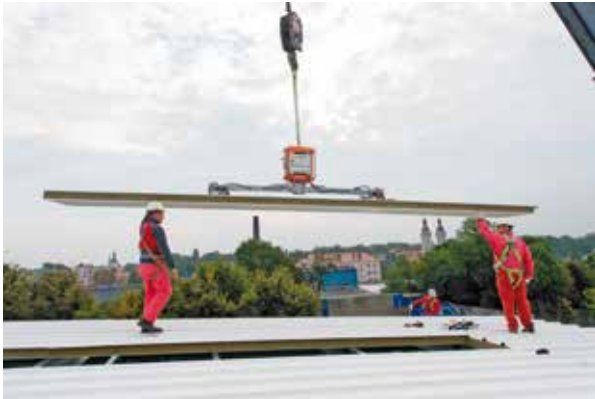
Pic. 8 and 9. Assembly of roof panels.
