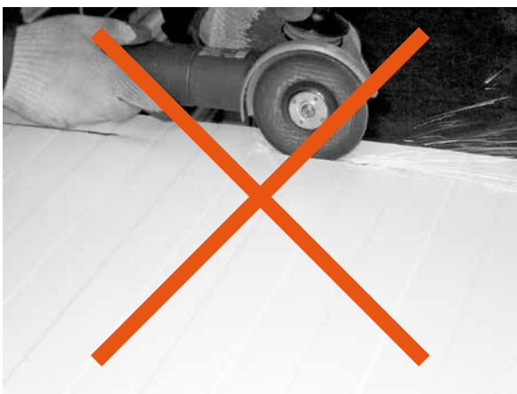
Pic. 6 and 7. Do not cut panels with angular grinding machine as anticorrosive covers can be devastated.
